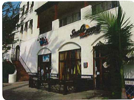
Figure 2.4.6 Stucco is effectively used in many architectural styles as an exterior wall material in Rivertown
