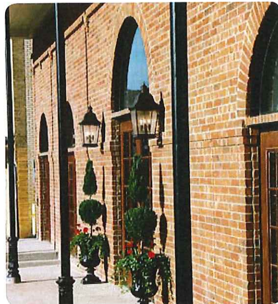
Figure 2.8.3 Doors are an integral part of a building's appearance and design
