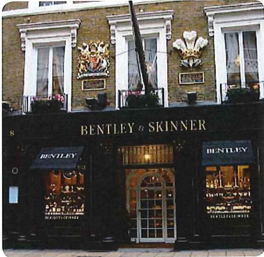
Figure 2.8.1 Storefront renovations complement the original design and materials for integrity
