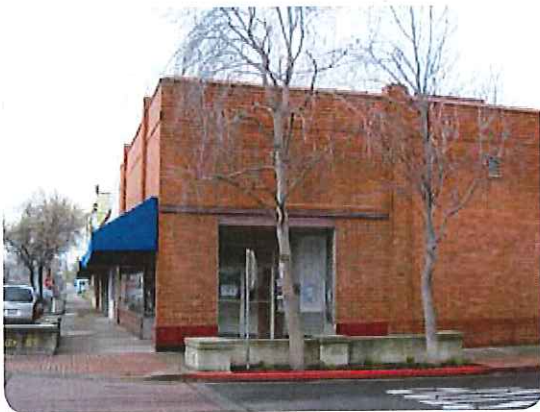
Figure 2.4.10 A typical flat roof commonly seen in Antioch
