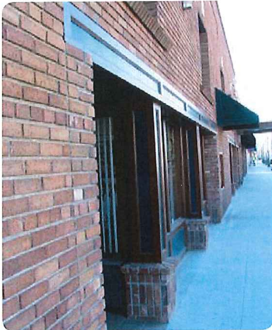
Figure 2.4.5 Minimizing the number of wall materials on a complex design enhances visual unity of design components
