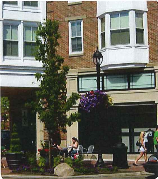
Figure 2.4.3 Bay windows provide vertical and horizontal articulation
