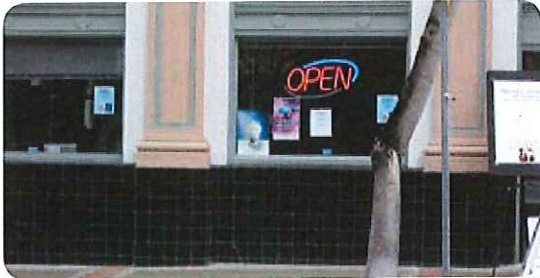
Figure 2.4.7 Tile used for bulkheads on the bottom of storefronts adds color and interest
