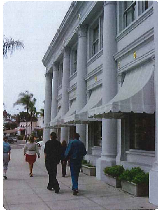
Figure 2.8.5 Paint can provide a fresh appearance for an older building's facade
